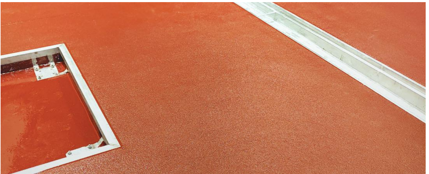
New plumbing- , a new drain system and a complete new pitching to the drains
